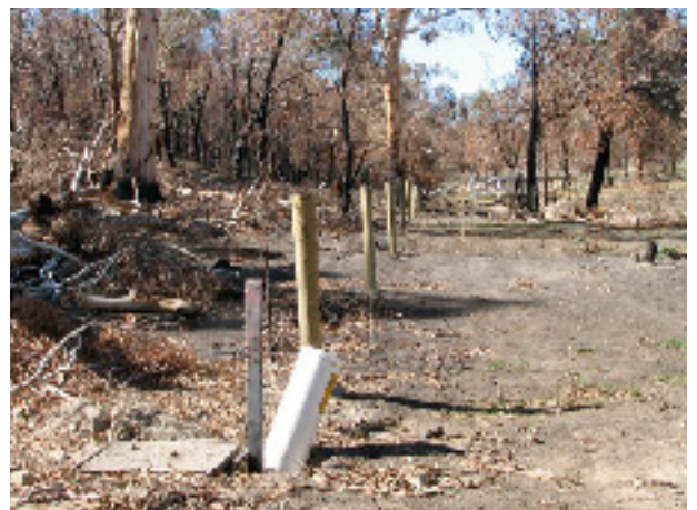
Some pine posts in place and waiting for re-wiring.
